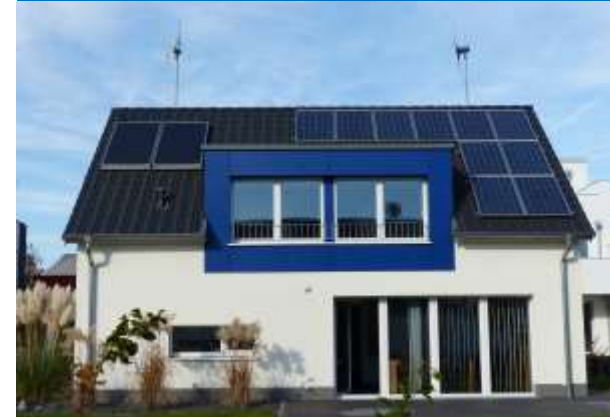
Decoupled towers mounted under the roof-tiles
