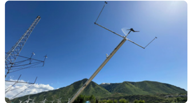
Stand-alone installation on a tower
