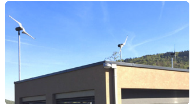
Flange-mounted to a flat roof building
